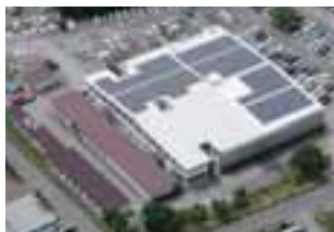
Solar panels installed on the roof of the Asama Plant
