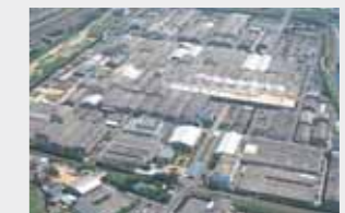
Chita Plant Address: 1, Maegata-cho, Handa, Aichi Major products: Insulators, equipment for electrical transmission and distribution, ceramic products for the chemical industry, beryllium-copper strips, ceramic components for semiconductor manufacturing, etc.
